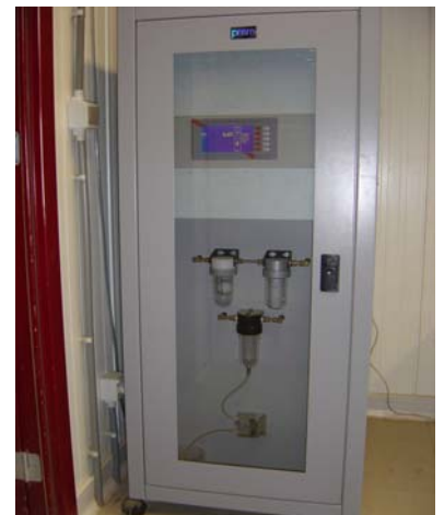
Ambiant CH 4 analysis Based on MGA3000 analyser CH 4 analysis Indoor or Outdoor Cabinet with gas sampling
